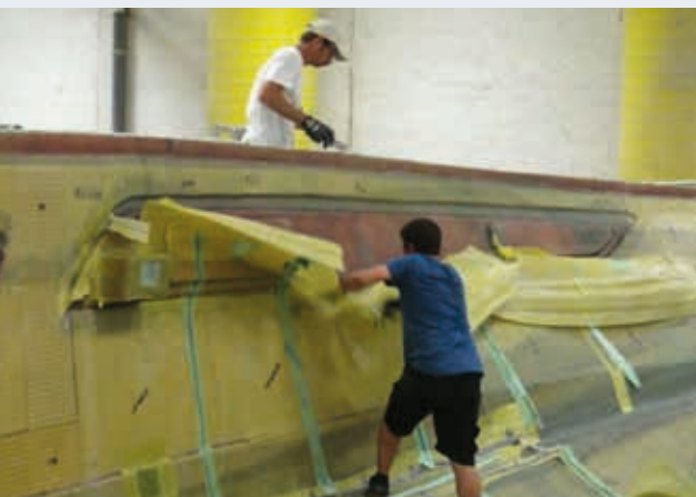
11. Minimum resin dust when removing Compoflex® RF 3.
