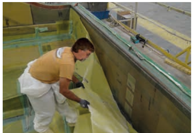
12. Minimum resin dust generated when peeling Compoflex® RF 3.
